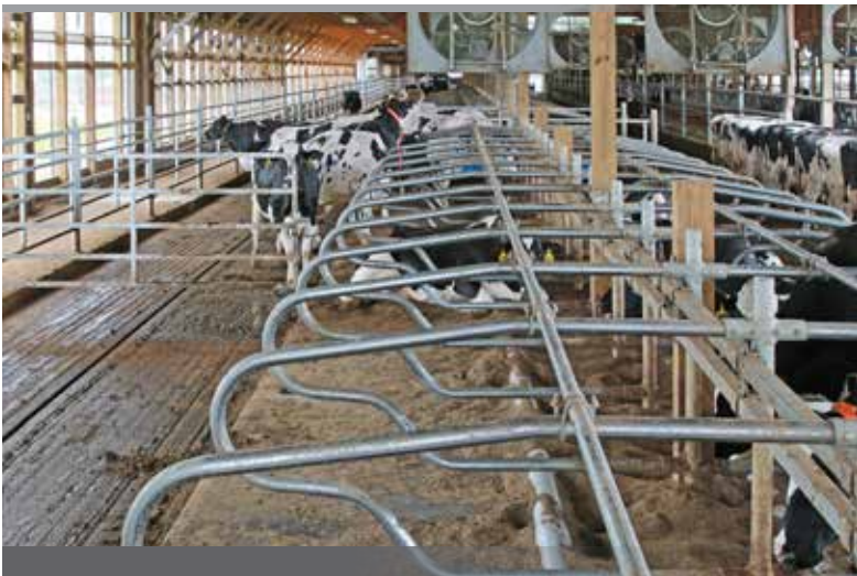
4-Bend Liberty Loops | Freedom Suspension to Wood Support Posts
