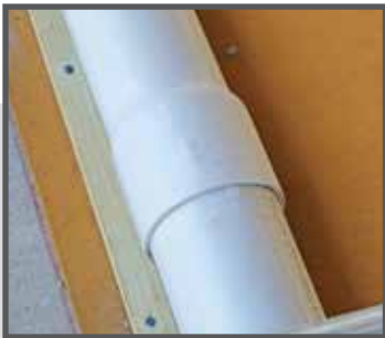
5" PVC Brisket Pipe (Bell End Connections)
