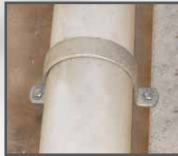
Double Tab Floor Mount Bracket
