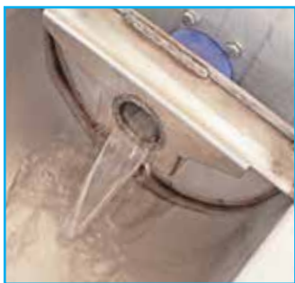
Fresh Water Supply
